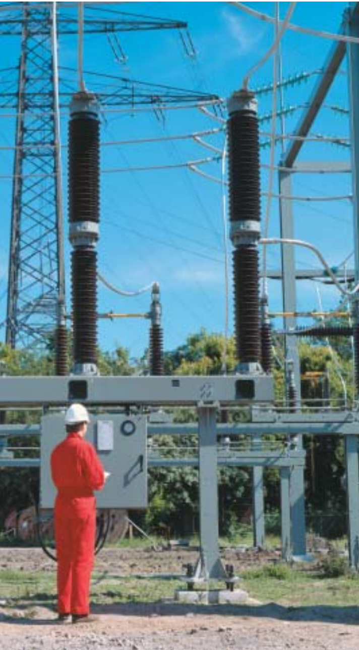
3AP1 FG 145 kV Live-tank circuit-breaker
