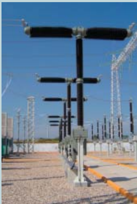
3AP2 FI 420 kV Live-tank circuit-breaker in operation at a major power transmission and distribution company
